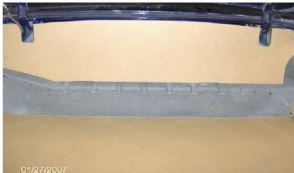
Note there is no dip in the center of floor panel. If you put weight in the panel then you will need to add support by using 2X4's.
