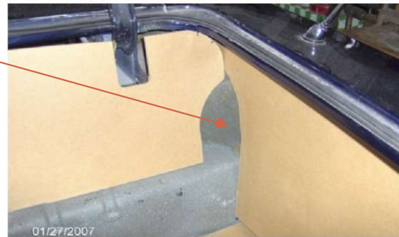
5. Test fitting is needed to insure proper clearance once material is added to the panels. Minor sanding with 80 grit will achieve proper fit.
